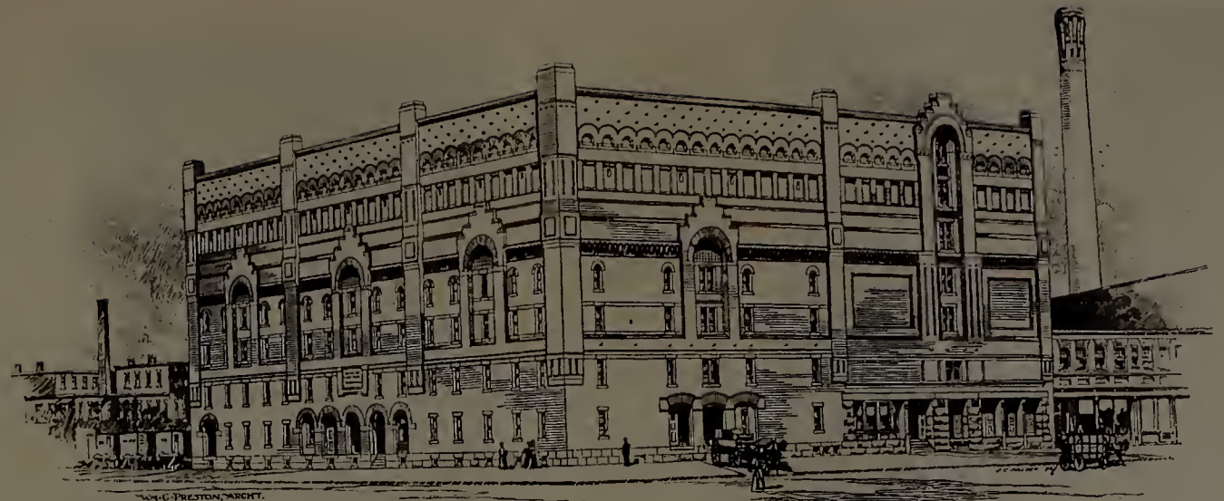
QUINCY MARKET COLD STORAGE COMPANY'S CENTRAL PLANT, corner of Richmond and Commercial Streets.
